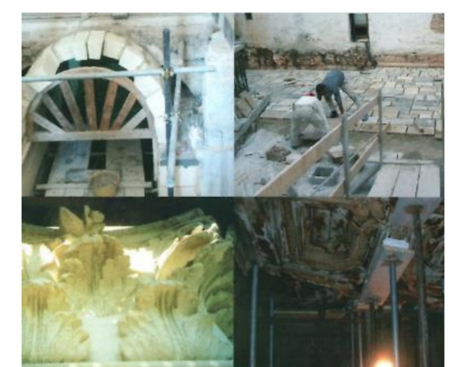
Embedding of the sensing element during the restoration
